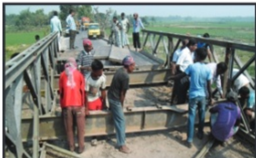
The workers are repairing the bridge.
