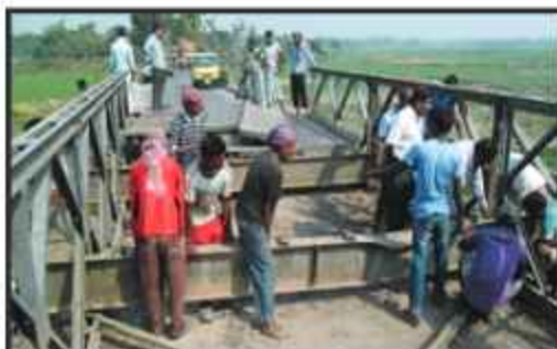
The workers are repairing the bridge.
